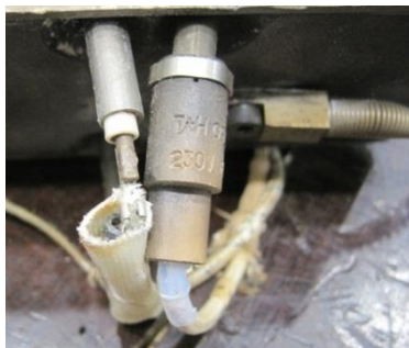
Figure 92: Unprofessional wiring
