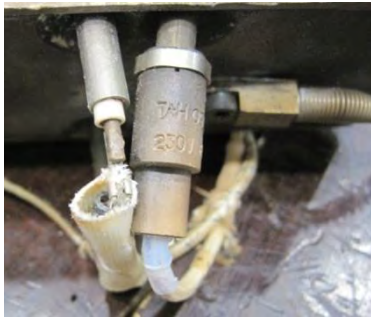
Figure 92: Unprofessional wiring
