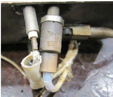
Figure 74: Unprofessional wiring
