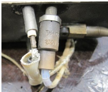
Figure 92: Unprofessional wiring
